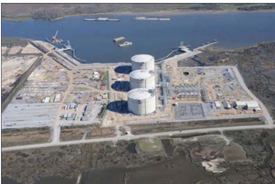
An aerial view last year of Sempra LNG's Cameron, La., terminal shows the site well along toward completion in late 2008 or early 2009 (Fig. 4; photo from Sempra LNG).
